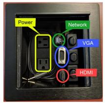
Laptop connections are in the cable cubby (Metal box in the AV cabinet directly under the control panel)
